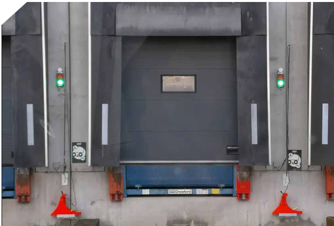
POWERCHOCK 3 installed and ready to be utilized.
