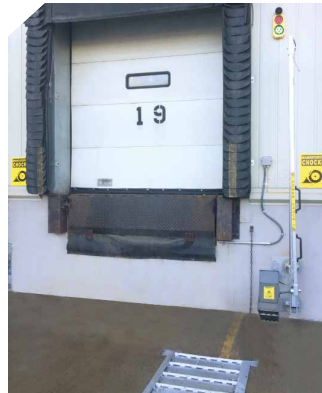
The winter adapted restraining plate of POWERCHOCK is a key element to cope with the snowplowing in colder regions.
