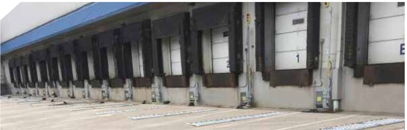
A LONG-TERM PARTNERSHIP | Some of the 49 doors at the SYSCO facility in Pittsburgh, PA.
